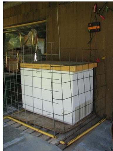
Figure 4 and 5. Electrified fencing used to permanently secure a hobbyists beehives near Libby and an outdoor freezer in the Yaak.
